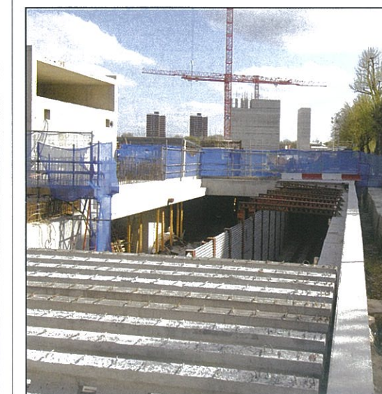
The eastbound running line of the Central Line is in the centre of this picture, with the access line to the new sidings to the left. This will all be covered over. Brian Morrison
