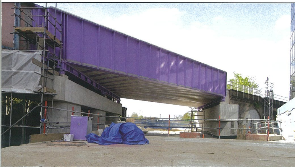
Below: New bridge for the Hammersmith & City Line. The access line to the new Central Line sidings runs under here. The entrance for the new H&C station for the shopping centre will be here, with platforms on the brick arch to the right. Wood Lane is to the left, and White City station on the Central Line is 200m away in the distance.
