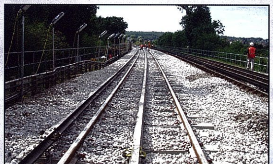
Taking shape: A new section after first pass of the tamper which puts track into the correct line and level
