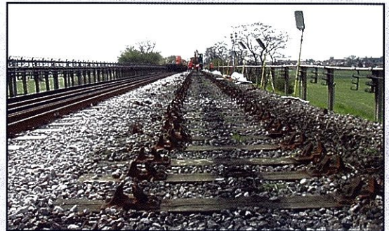
Work gets under way: Between Fairlop and Barkingside, rail removed
