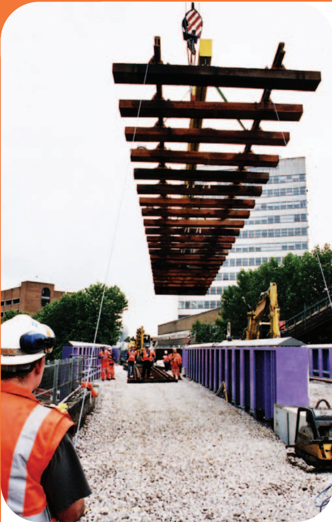
Track being laid.
