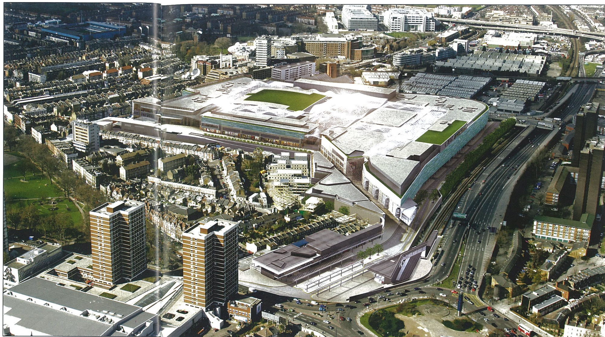
Impression of aerial view of the finished development. The West London line runs down the right hand side of the development, with the new station at the bottom of the picture adjacent to the remodelled Shepherd's Bush Underground station.
